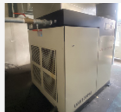
Inverter Compressor Replacement
